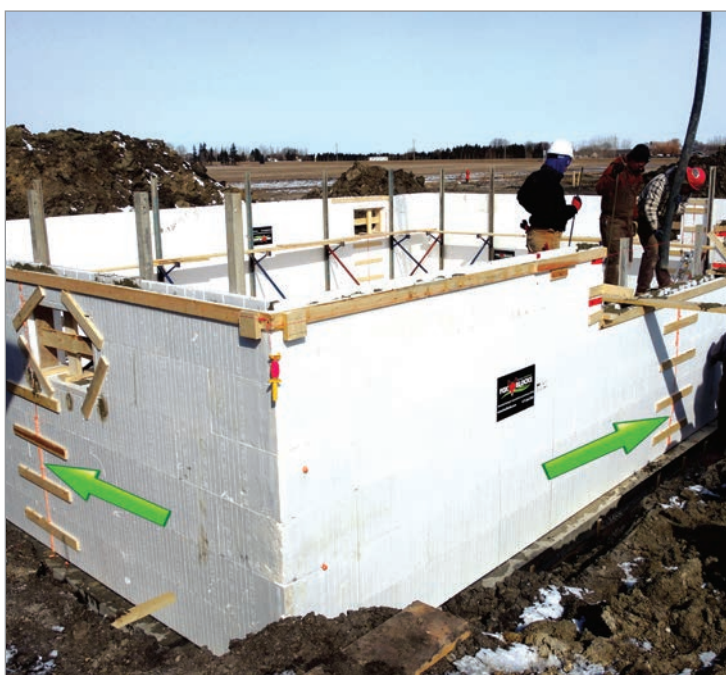
Here is a job, post concrete, that has been constructed exactly to the building dimension by properly stacking seams.
